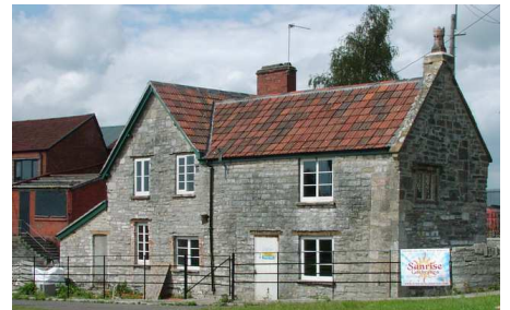
Northover Mill, from 1517, is the first building in Glastonbury seen by visitors from the M5.
