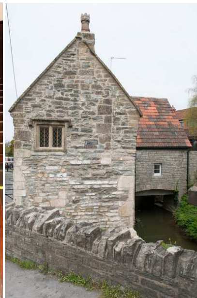
Left: Fine woodwork in the office part of the Baily tannery. Right: New leaded-light windows at Northover Mill. The effectiveness of its new heat-exchange system impressed visitors: energy is extracted from the water passing beneath the building. The system is cheap to run, though expensive to install. (Photos by David Thomas)
