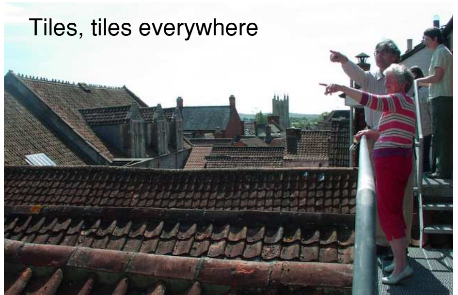
The roofscape between the High Street and the Abbey ruins was a fascinating aspect of the tour of Burns the Bread which Conservation Society members enjoyed on June 1. Maggie Stewart, Adrian Pearse and Debbie Fear here are standing on the fire-escape behind the bakery's upper floor, the Assembly Rooms are at left and the tower of St Benedict's Church in the distance. One wall at the back (off the left of photo) might be pre-Norman; Neill Bonham thinks it was part of a building that was old even in Abbey times.
