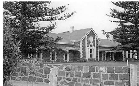
James Austin built Avalon Homestead, on Corio Bay near Geelong (about 35 miles southwest of Melbourne). After a fire in 1870, a nephew rebuilt the single-storey house in basalt and freestone. A carved Tudor rose from Glastonbury Abbey, which James by then owned, is set into the covered entry. Bluestone stables for the Austin racehorses stand behind the house. The land remained in Austin hands for many years but is now subdivided; part is now Avalon Airport. Avalon College, a boarding school for Asian language students, took over the house in 1998.
